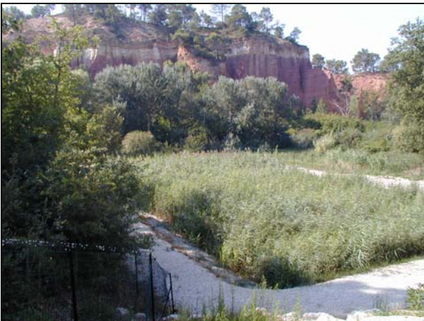
Phragmifilter® Wastewater treatment plant of Roussillon (84) – 1200 p.e. –
