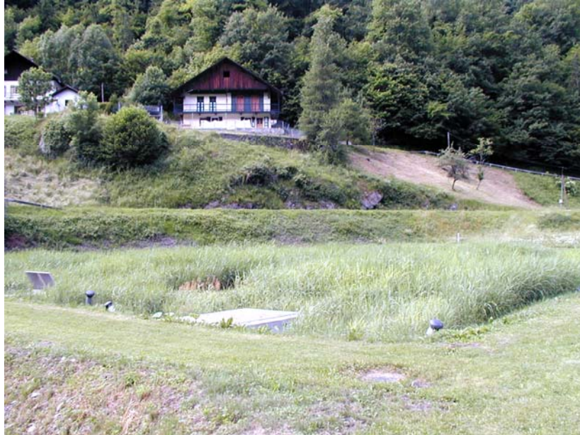
Queige (73) – 500 p.e. – Phragmifilter® wastewater treatment plant
