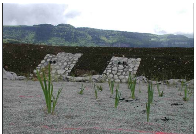
Neydens (74) – storm water retention and treatment
