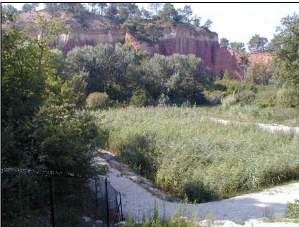
Phragmifilter® Wastewater treatment plant of Roussillon (84) – 1200 p.e. –
