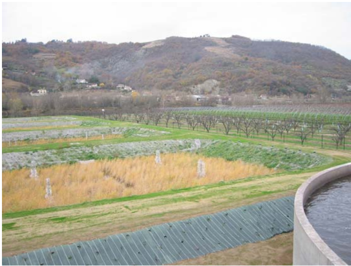
Reed beds for sludge treatment
